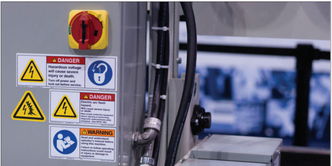
Figure 3: Example of a symbol-only label with the new arc flash symbol placed next to an arc flash safety label (Label designs ©Clarion Safety Systems. All rights reserved.)
