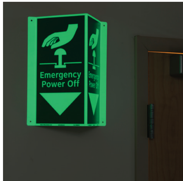
Figure 4: Example of a photoluminescent emergency stop button safety sign mounted in a facility
